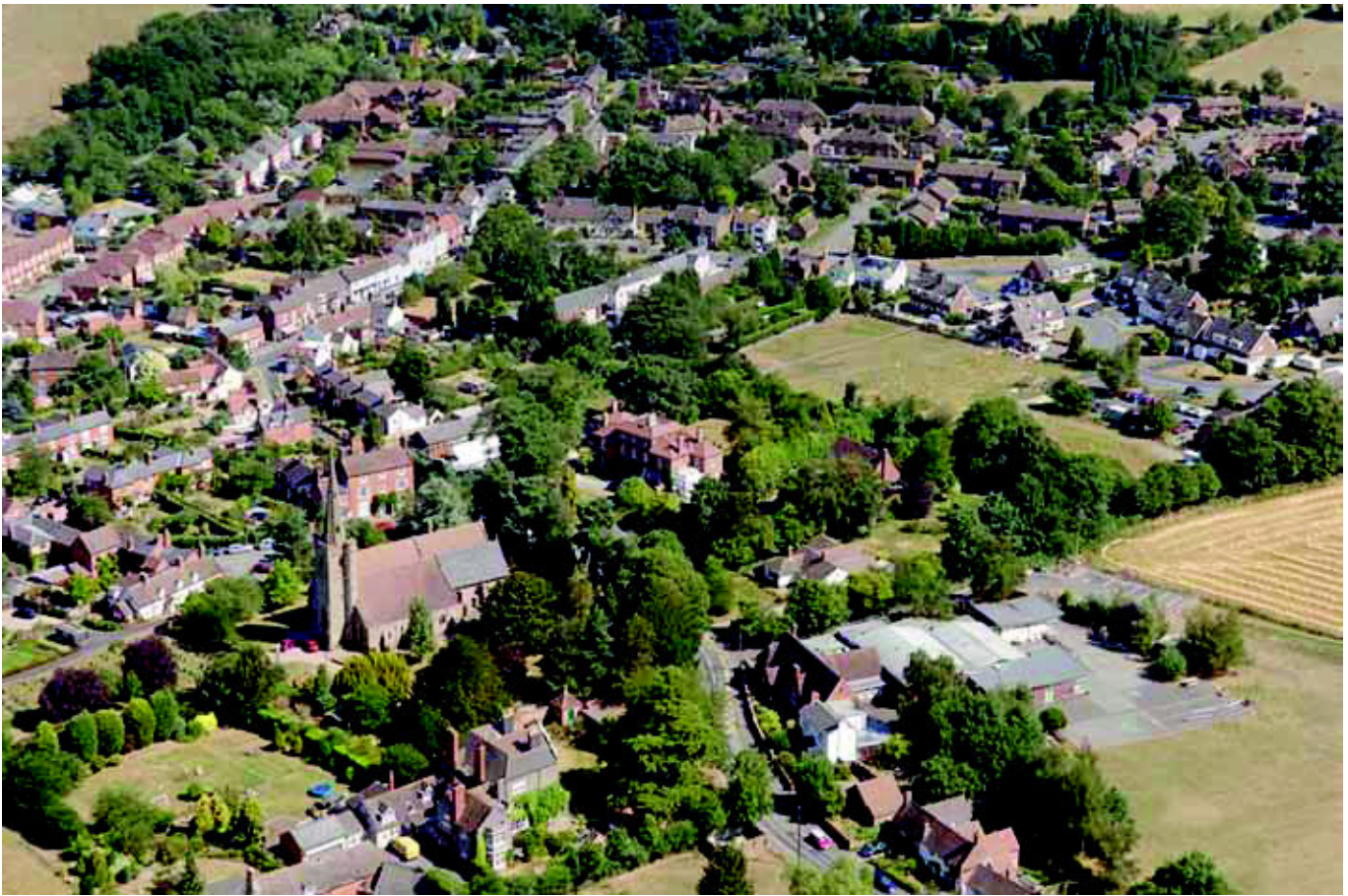
Aerial view of Belbroughton
